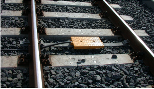
Figure 4. ETCS Eurobalise installed on the track see https://en.wikipedia.org/wiki/European_Train_Control_System , CC BY-SA 4.0
