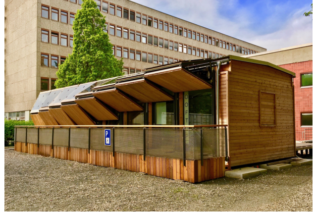
Figure 4. Rooftop building with roof and facade mounted photovoltaic system in Berlin (Germany).
