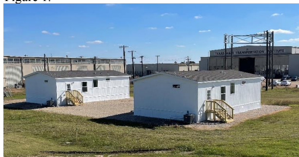
Figure 1. The Texas A&M Smart and Connected Homes Testbed (TAM-SCHT)
