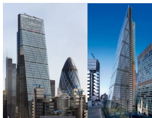
Figure 2: The Leadenhall Building ( right photo: (Esper, 2007), and the left photo: (Howarth, 2014))
