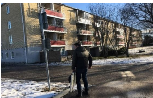
Figure 6: Test installation site
