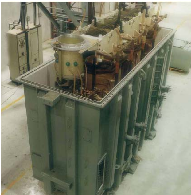
Figure 1: Model of heat generation and transfer in power transformer in the above and so tank and windings&cores of power transformer, in the below.
